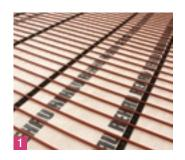
Underfloor heating is increasingly being specified over traditional radiator systems as the preferred modern-day heating solution.
