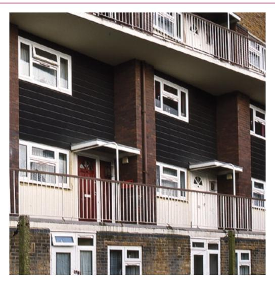
No longer restricted by traditional fire rated materials and construction techniques, RAUFERNO gives you the freedom to use PVC-U fire resistant windows and fire resistant doors and still comply fully with 2006 Building Regulations for most protected areas, due to full certification to BS 476 Parts 20 and 22.
