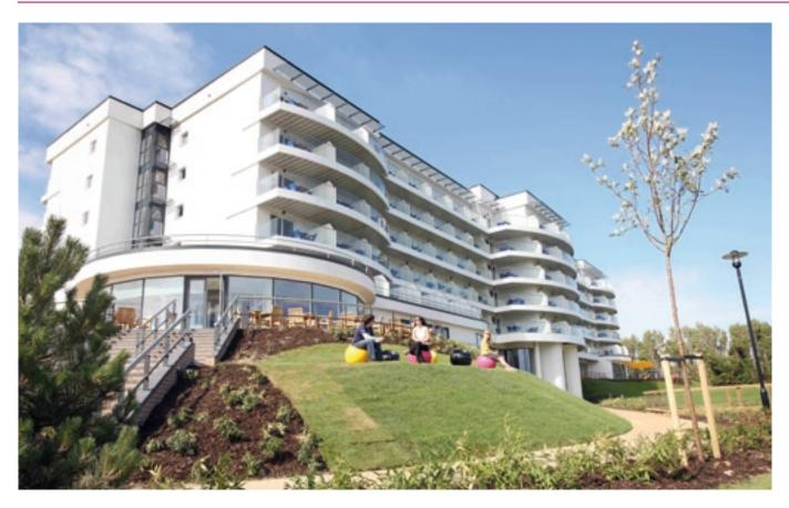
Composite curtain walling system REHAU Polytec 50S combines the benefits of Aluminium, Steel and Polymer materials providing an outstanding thermal performance with an  $U_f$ -Value of up to 0.88 W/m<sup>2</sup>K.
