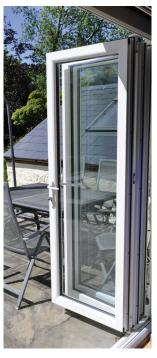
A frame rebate filler is available to provide colour match in the rebate if required.
